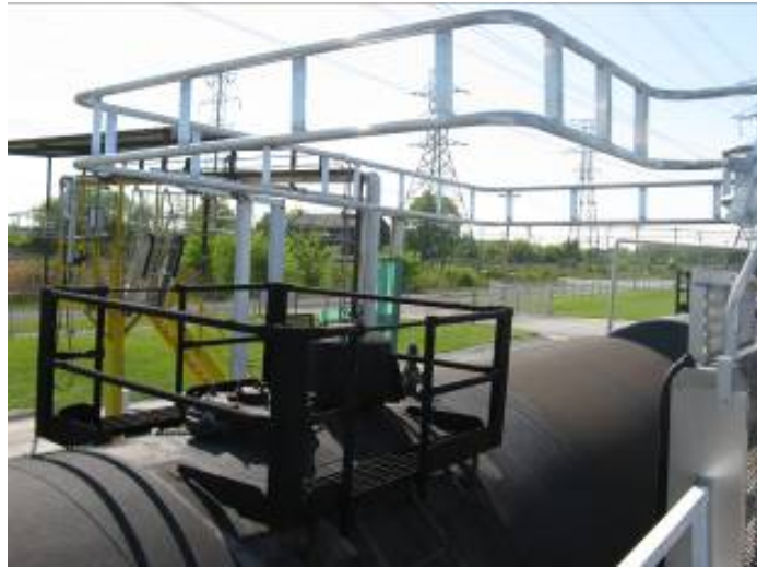
Figure 11: Small Work Platform, Large Cage
