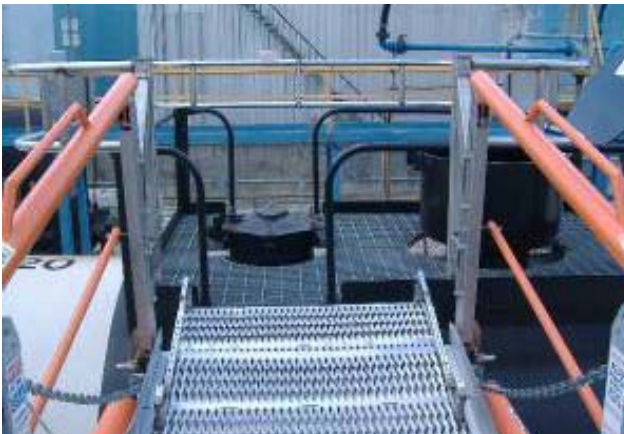
Figure 9: Large Work Area, Gangway and Smaller Cage
