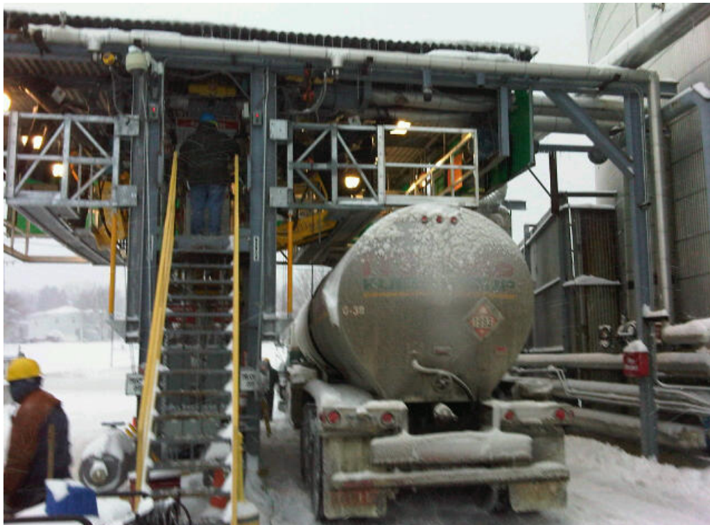
Figure 3: Truck Rack Retrofitted with Gangway, Platform and Cage
