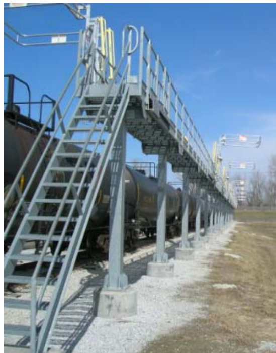
Figure 13. Newly Constructed Railcar Access Platform with Retractable Gangways and Cages
