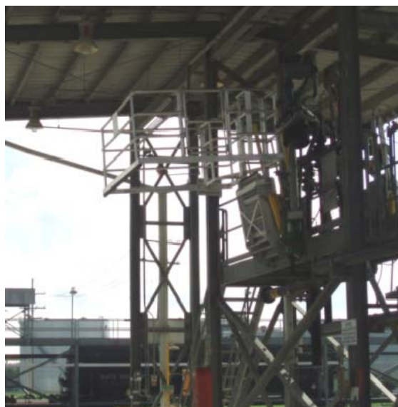
Figure 4: Truck Rack Retrofitted with Gangway and Cage
