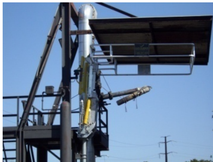
Figure 5: Rail Loading Platform Retrofitted with Gangway and Cage
